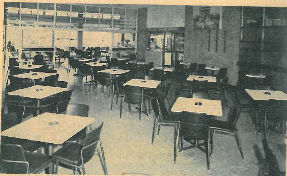
The ground floor lounge/dining room extends from the front of the hotel through to the parking area at the rear.
